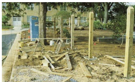
Merely identifying trees to save on a site plan is not sufficient. It is critical that tree professionals be an essential part of the development team on any project. Here, no effort was made to defend tree resources and tissues. (Photo courtesy of Kim Coder)
