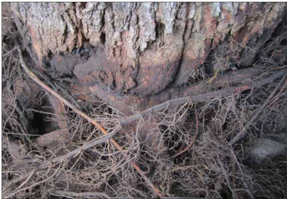
Fibrous epicormic roots can generate rapidly from damaged cambial tissues if mulch and amended soils are placed in direct contact with the excised roots and trunk tissues after girdling roots have been removed.
