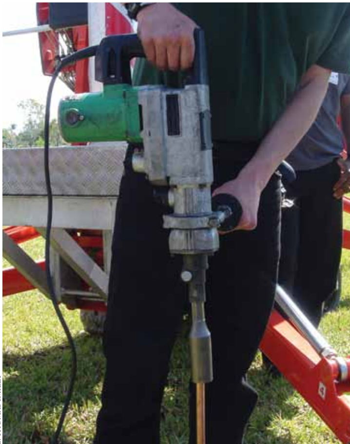
Figure 7. Ground rods must be no less than one half-inch (13 mm) in diameter and eight feet (2.4 m) long. The typical ground rod has a steel core for strength and is clad in copper for conductivity and corrosion resistance.
