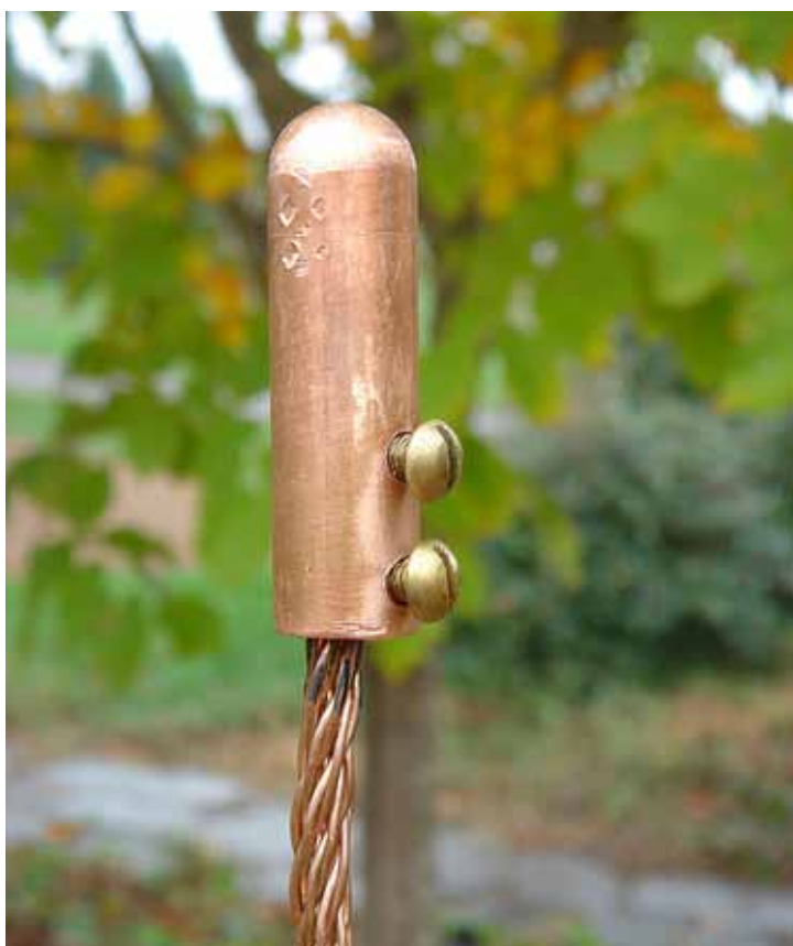
Figure 6. A tree lightning protection system is not required to be terminated with a manufactured air terminal, but the use of a manufactured blunt air terminal is preferred because they are more effective at attaching the strike to the TLPS.
